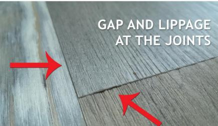
If the long edge of the plank is not fully engaged and a small gap is left, the short side will not click into place as you see in this picture. You will feel the lippage on both joints. When you are engaging the short side, use a small rubber mallet and a scrap piece of plank to spread the force. Check your work to make sure that both the long side and the short side is fully locked and that there are not gaps, before you continue to the next row.
