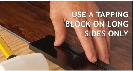
With each plank, inspect your installation and check for gaps. The gaps might be very tiny, so use a taping block on the long sides to close them. Working against a wall that is not straight will cause gap problems. Watch the video on the next page for a solution.
