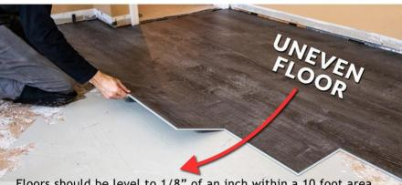
Floors should be level to 1/8" of an inch within a 10 foot area.
